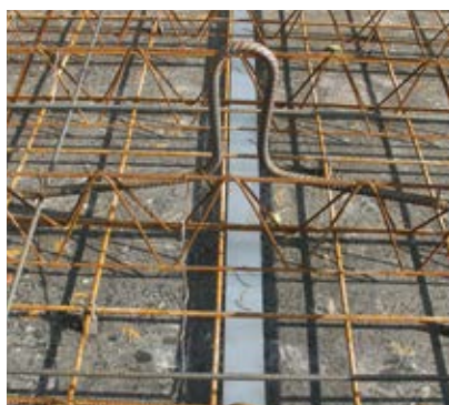
④ INSTALLATION RENFORCEMENT
