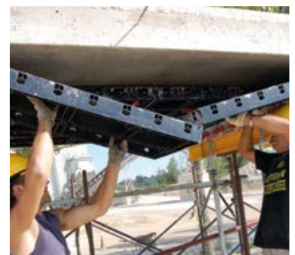
⑧ DEMONTAGE: GEOPANEL
