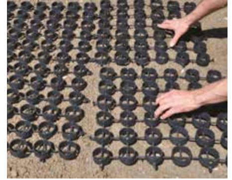
③ INSTALLATION GEOGRASS installation.
