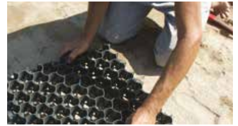
③ INSTALLATION Installation of SALVAVERDE that guarantees the drainage of rainwater and the protection of the turf.
