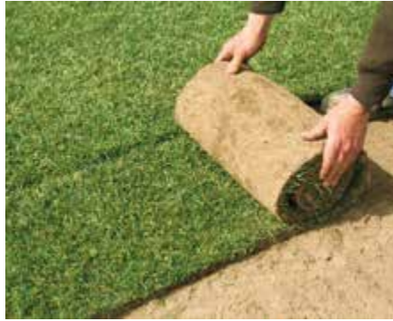
⑤ SEEDING Grass seeding and installation of the roll of sod.
