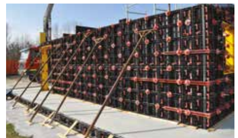
SHORING BEFORE PLUMBING
