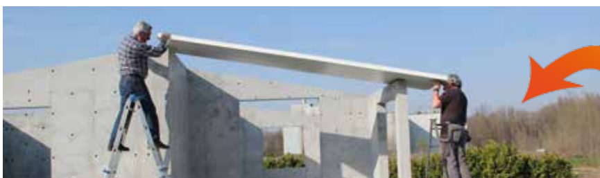
ROOF AND FRAMES INSTALLATION
