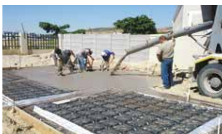
SINGLE POUR OF CRAWL SPACE AND FOUNDATION BEAMS
