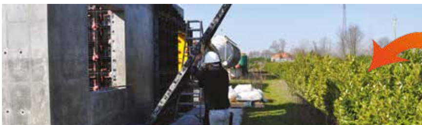
WALLS FORMWORK DISMANTLING
