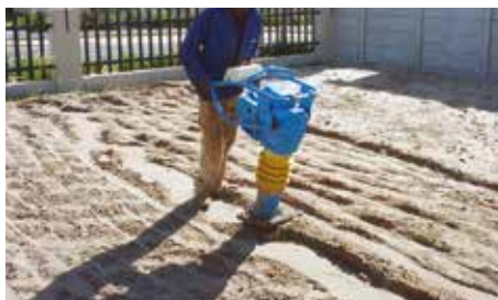
FOUNDATION TRACING AND SOIL COMPACTION
