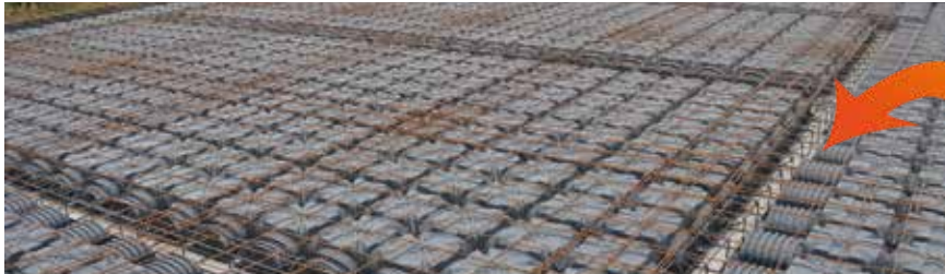
CREATION OF THE FOUNDATION SLAB
