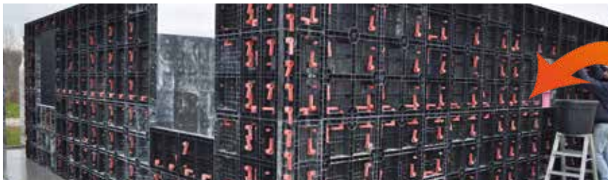
WALLS FORMWORK INSTALLATION
