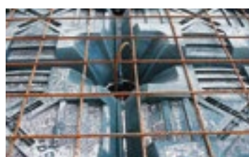
Reinforcement of the pillar with steel forks
