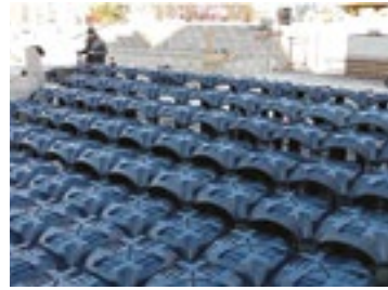
Detail of the formwork installation
