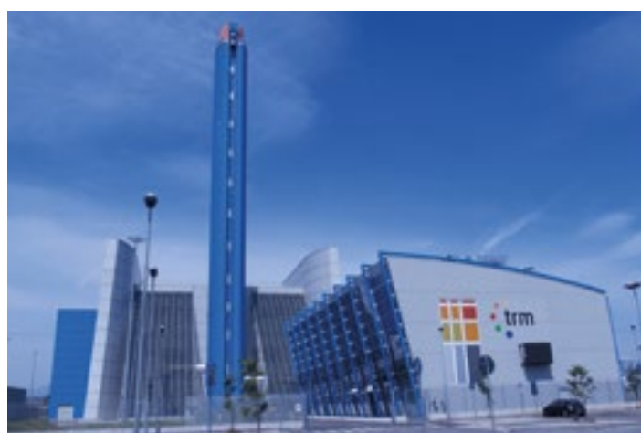
TRM Incenerator, Italy
